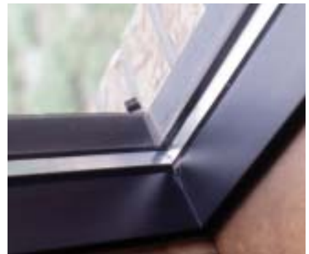
Aluminum that is exposed to the elements can be anodized to enhance the naturally occurring oxide that forms on its surface and to protect the base metal from attack by atmospheric components.
