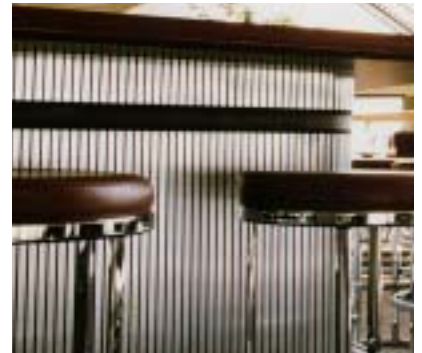
Anodized aluminum is aesthetically pleasing as well as durable. Here it is used as a decorative element in a restaurant bar area.
